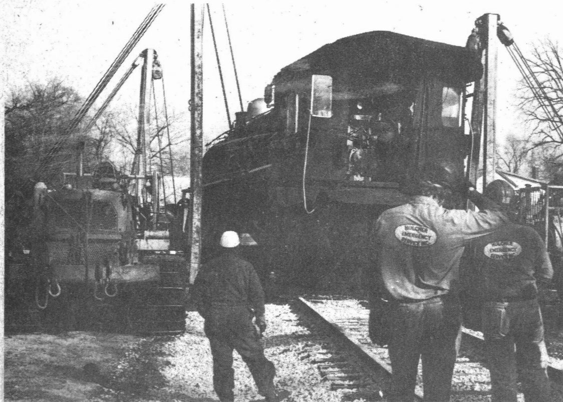
Rail Alignment At Rail's End
